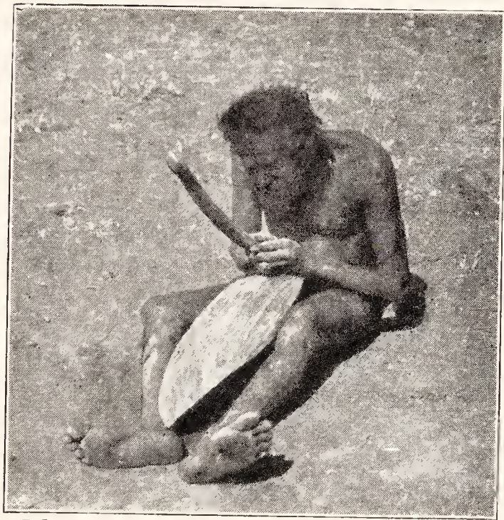
FIG. 349.—MAN USING ADZE FOR MAKING THE GROVES ON THE OUTSIDE OF A PITCHI, WARRAMUNGA TRIBE.
