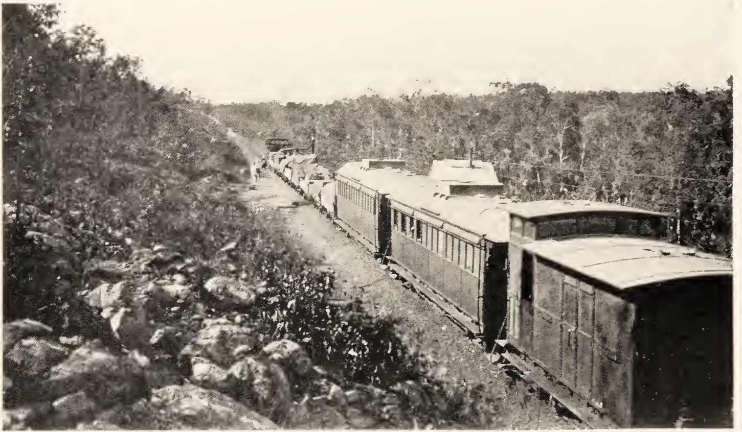
FIG. 491.—WAYSIDE STATION ON DARWIN-PINE CREEK RAILWAY.
